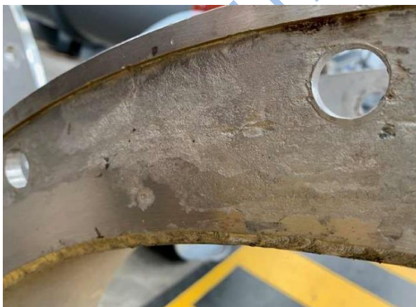
Figure 5-2 Crevice corrosion of 316L (© Roger Francis)
